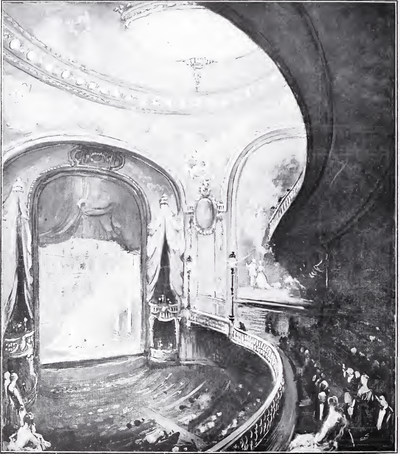
THE RECONSTRUCTION OF THE AVENUE THEATRE, LONDON.
