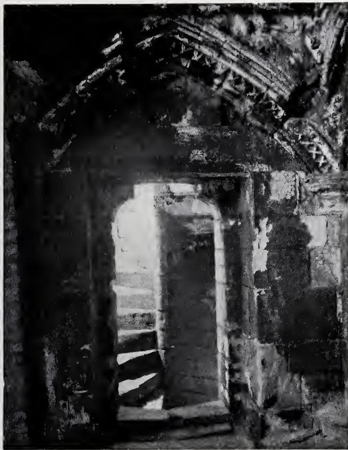
STAIRCASE, CLIFFORD'S TOWER, YORK.
