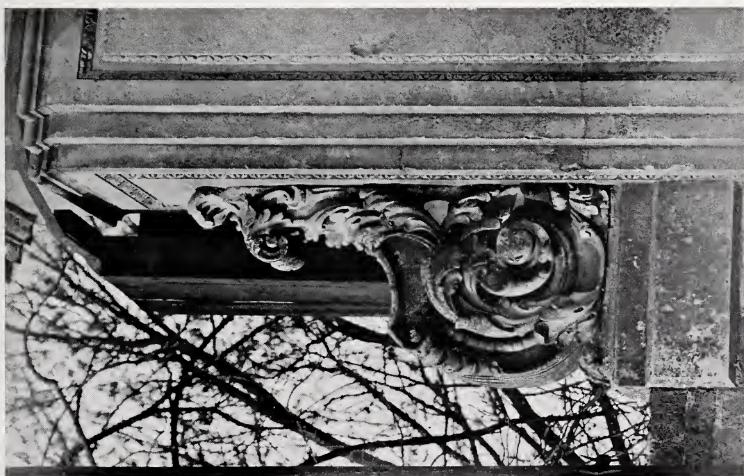
Detail of bracket. CARSHALTON PARK GATES.
