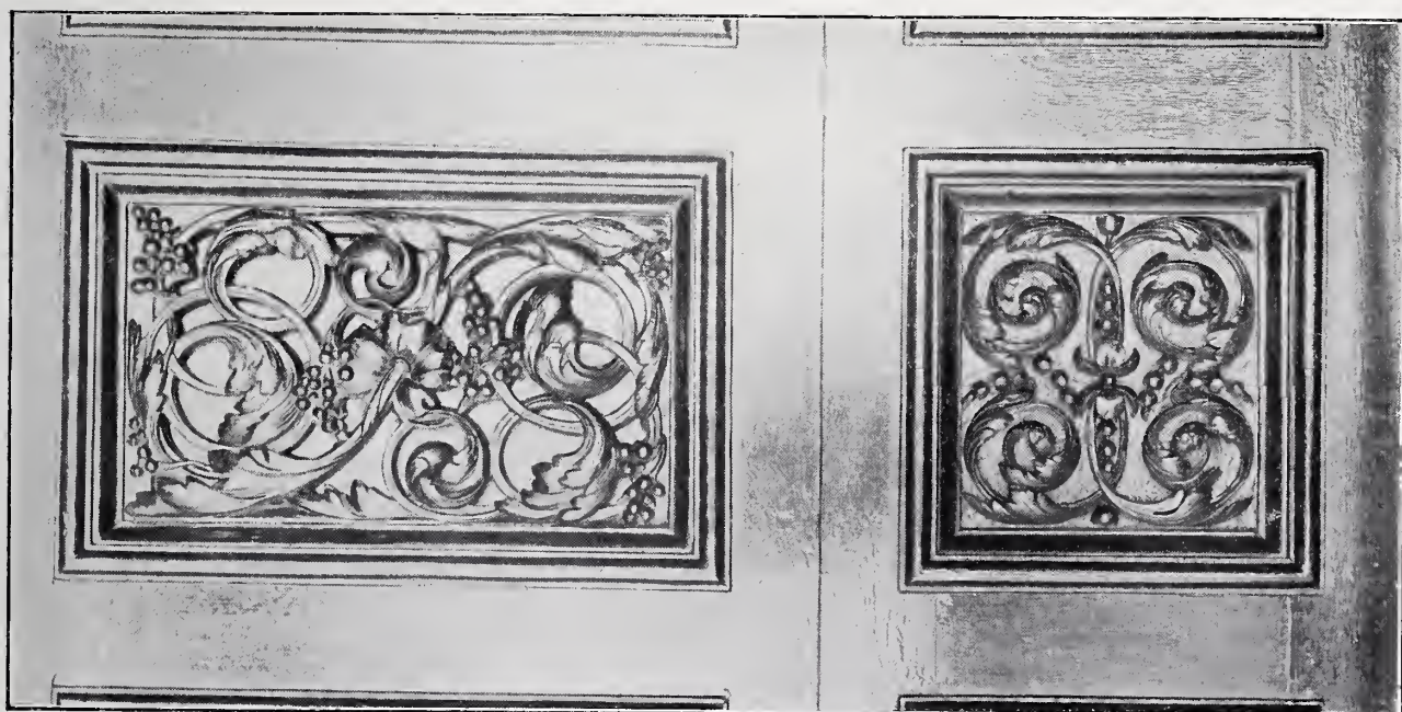
Detail View of Panels to Chapel Door.
