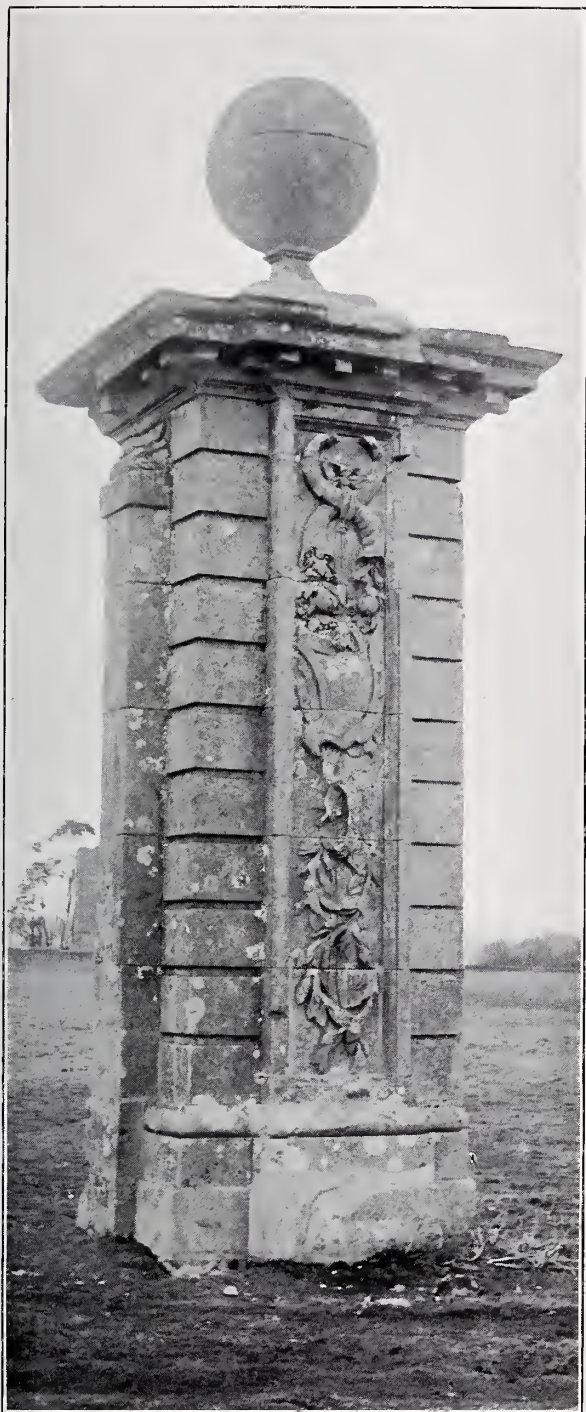
GATE PIER "B," HAMPSTEAD MARSHALL, BERKS. For measured details, see next page.
