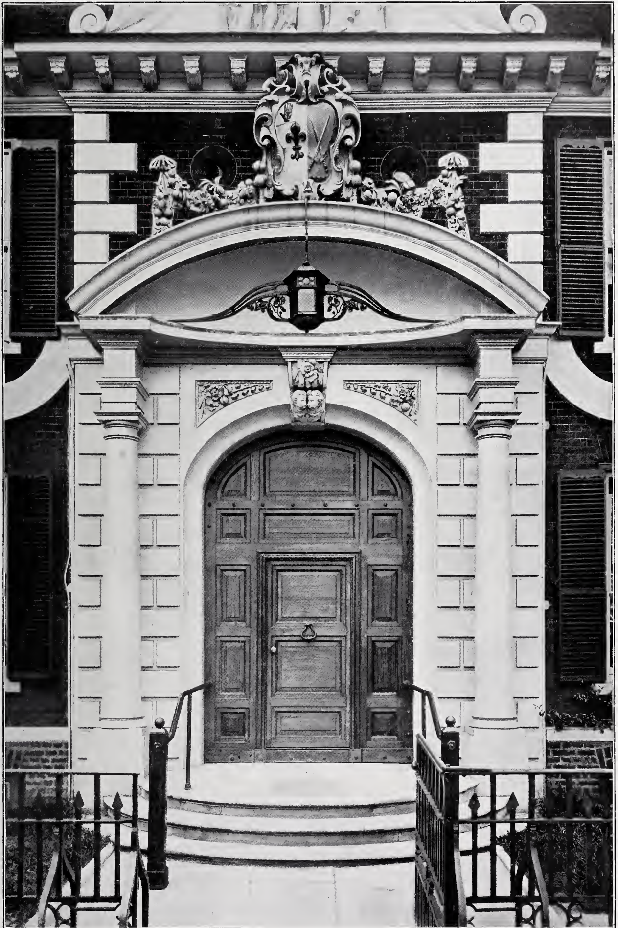
MORDEN COLLEGE, BLACKHEATH. MAIN DOORWAY.
