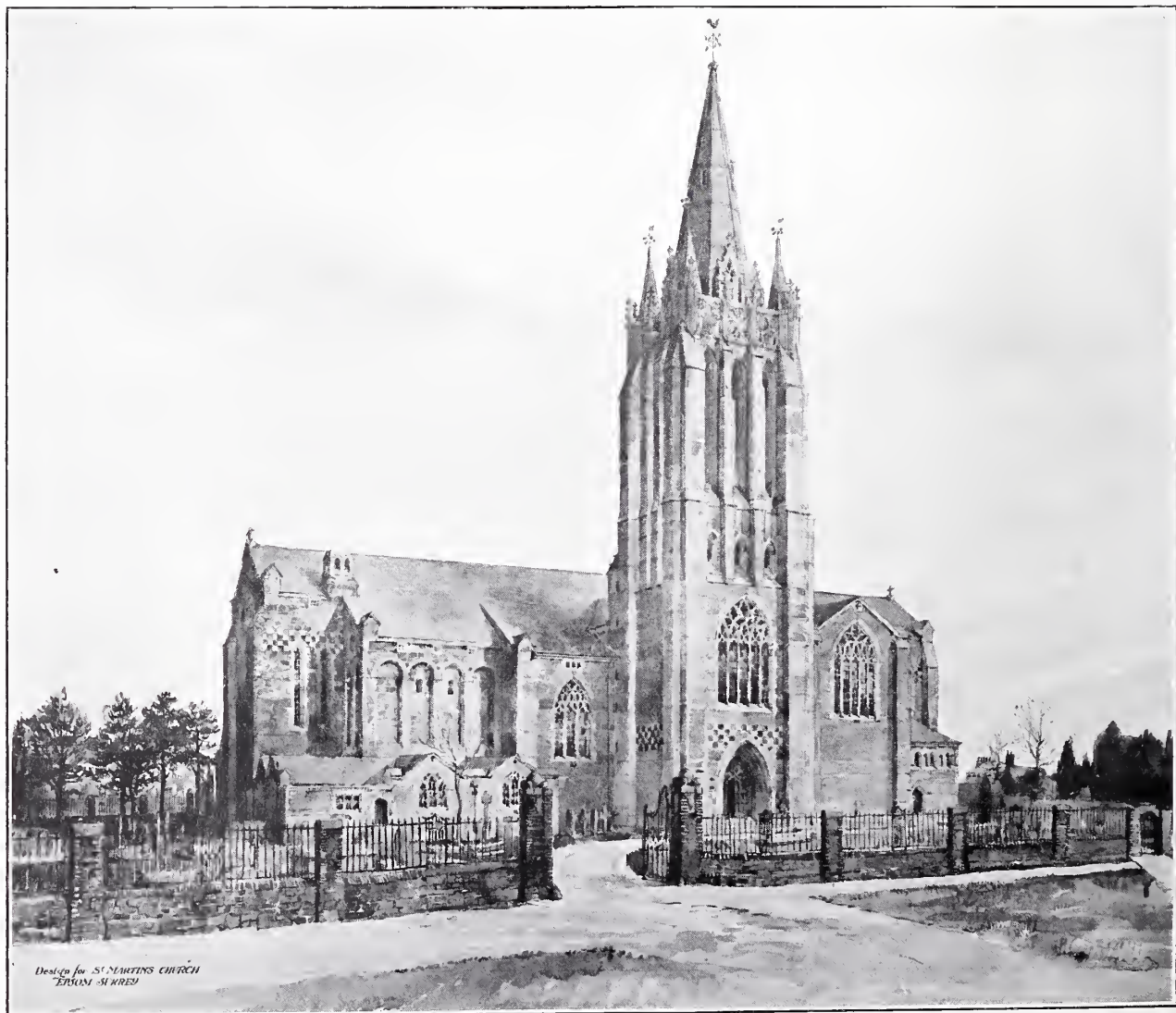
NO. 1515. NEW PARISH CHURCH, EPSOM. SIR CHARLES A. NICHOLSON, BART., ARCHITECT.
