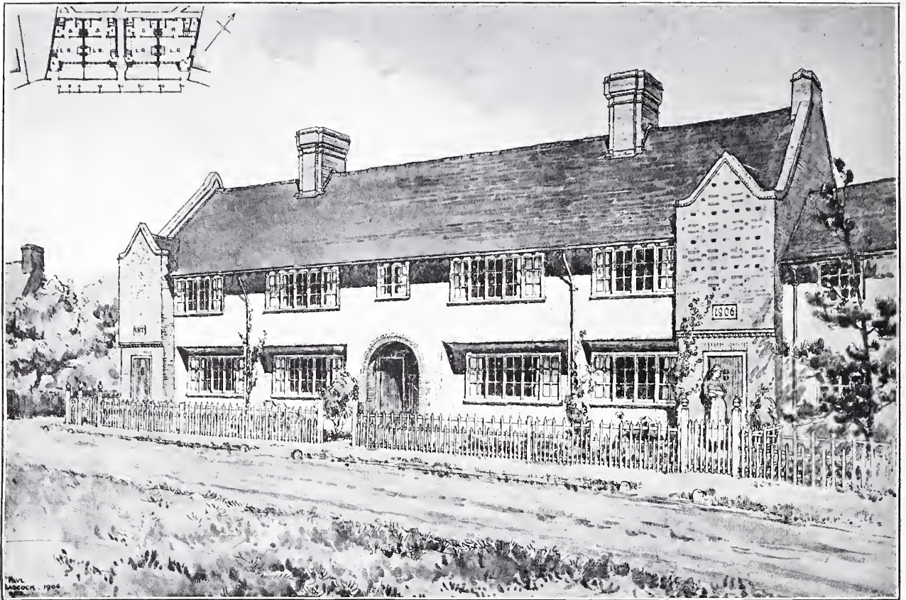
NO. 1452. COTTAGES AT SOUTH MYMS, HERTS. GEOFFREY LUCAS, ARCHITECT.
