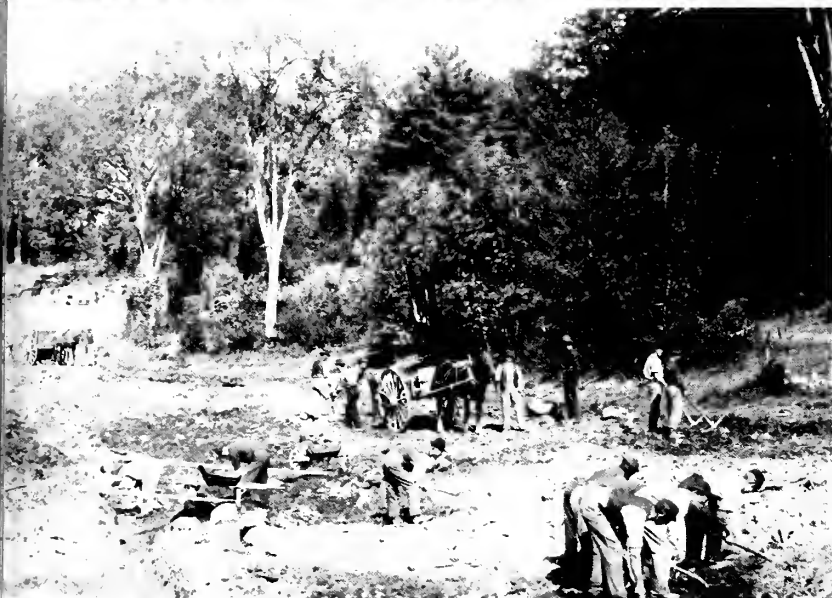
1 construction in the Arboretum began in 1883, and the plant families in permanent systematic collection were sited as the road work progressed. Top: photograph, taken in October 1890, shows the area around Lily and Bussey Ponds. Bottom: Construction of the roadway at the Walter Street entrance, 1899. Photographs by the Boston Park Commission.
