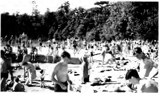
The swimming beach as it looked in 1948. This photograph, taken on July 11, 1948, by Roland Wells Robbins, shows the beach from the south, while Gleason's view shows it from the west. The slope in the background was denuded of trees and bulldozed in 1957 to enlarge the beach.
