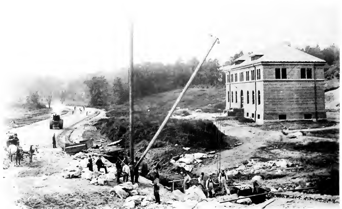
The Hunnewell Building under construction in 1892. All photos are from the Archives of the Arnold Arboretum.
