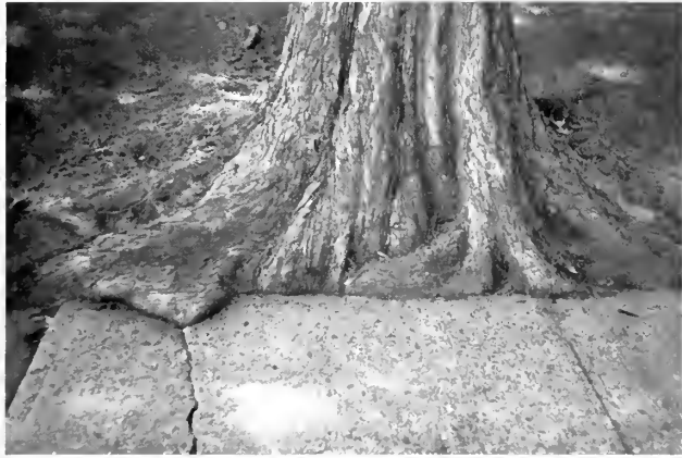
The roots of a dawn redwood planted too close to a sidewalk thirty-five years ago in Paramus, New Jersey.
