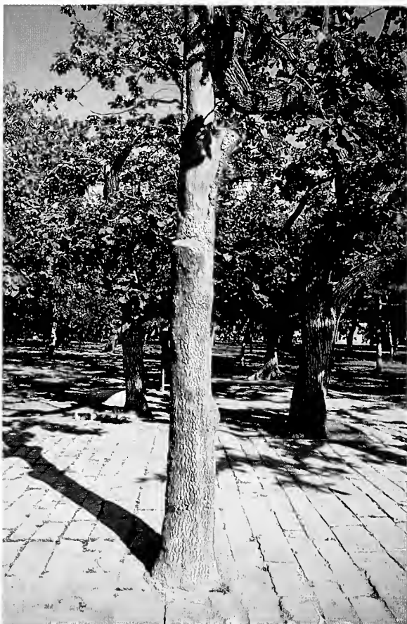
18: Tree support, concrete. Ming Tombs, Dingling, China, 2005.
