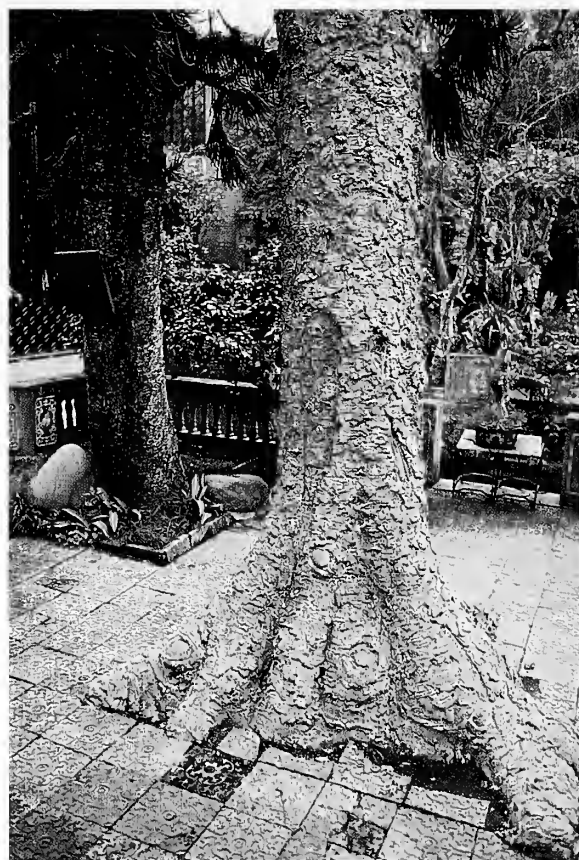
19: Tree support, Araucaria cunninghamia , concrete. Yu Yin Shan Fang garden, Panyu, Guangzhou, China, 2005.
