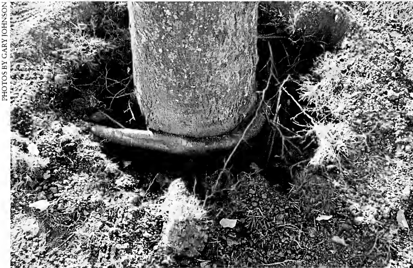
Figure 6. This SGR, located approximately 4 inches below ground, runs tangential to the tree trunk and is compressing 30% of the stem circumference.
