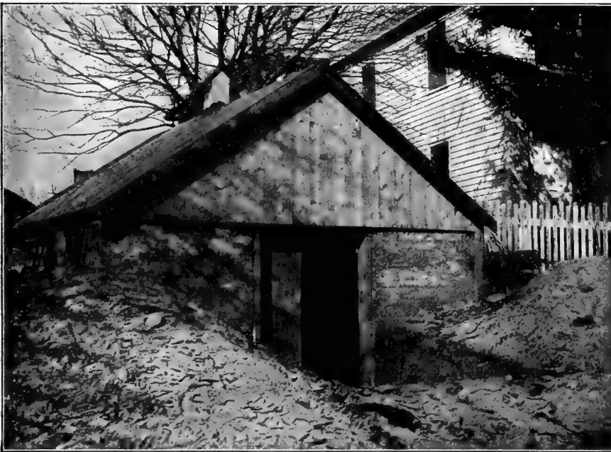
FIG. 100—CONCRETE INCUBATOR CELLAR
