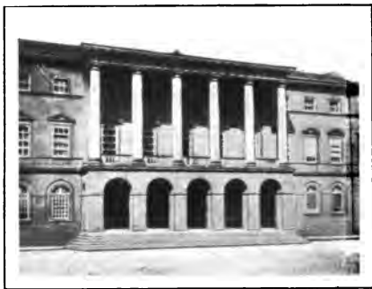
FIG. 673.—OPORTO. HOSPITAL OF SANTO ANTONIO. (Author's Phot.)
