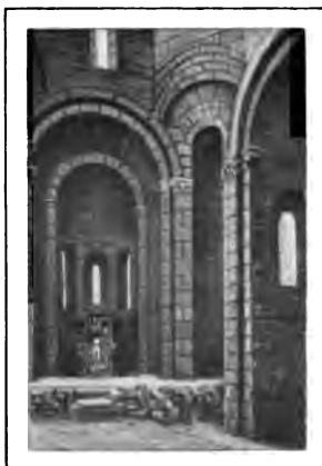
FIG. 73.—KARA KILISSA (Type \alpha ). CUPOLA ON SQUINCHES.
