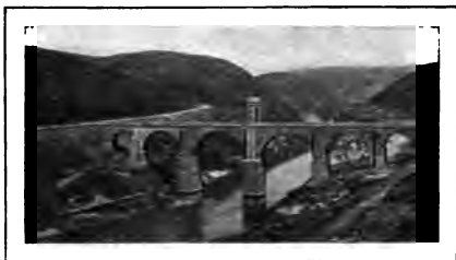
FIG. 101.—BRIDGE OF ALCANTARA. ( Phot. Lacoste. )
