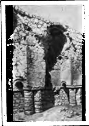
FIG. 23.—PALAIS DE SARVISTAN. GALLERY C ( vari. γ ). BARREL VAULTS, BUTTRESSES ON COLUMNS, SEMI-CUPOLAS ON SQUINCH ARCHES. (Author's Phot.)
