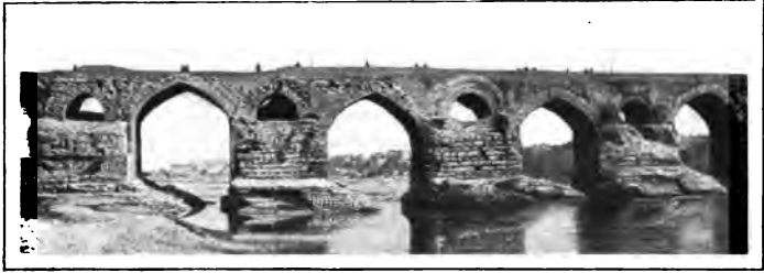
FIG. 36.—SASSANIAN BRIDGE OF DIZFUL. ARCHES RECONSTRUCTED. (Author's Phot.)
