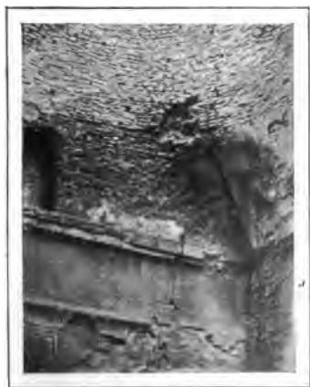
FIG. 18.—PALACE OF FIRUZ-ABAD. CUPOLA ON SQUINCH ARCHES OVER THE GREAT HALLS. (Author's Phot.)
