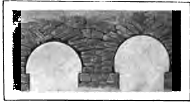
FIG. 82.—PALACE OF FIRUZ-ABAD. HORSE-SHOE ARCHES (INNER DOORS).
