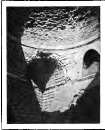
FIG. 27.—SARVISTAN. HALL A, CUPOLA ON SQUINCH ARCHES. (Author's Phot.)
