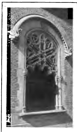
FIG. 433.—ALCALÁ DE HENARES. WINDOW OF PALACE. ( Author's Phot. )
