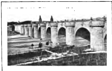
FIG. 538.—MADRID. TOLEDO BRIDGE.
