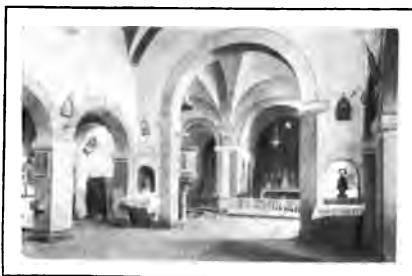
FIG. 111.—SANTULLANO. NAVE, AISLES, TRANSEPT, APSE, AND APSIDAL CHAPELS. ( Phot. Hauser y Menet. )
