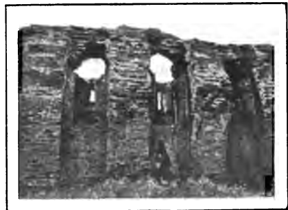
FIG. 30.—TAG-È IVAN. DOUBLEAUX (TRANSVERSE ARCHES), FORMERETS (LATERAL ARCHES), WINDOWS, SPRINGING OF MINOR ARCHES.
