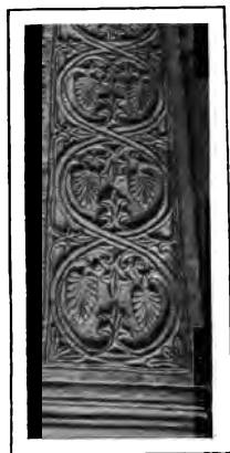
FIG. 170.—DECORATED LINTEL. WELL AT MERIDA. (Author's Phot.)
