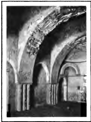
FIG. 25.—KASR KHARANEH. AT THE END OF THE HALL A SEMI-CUPOLA ON SQUINCH ARCHES.
