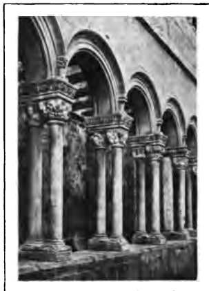
FIG. 151. RIPOLL.—TWO-STOREYED CLOISTER OF THE ABBEY CHURCH.
