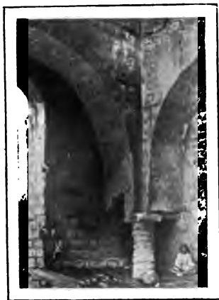
FIG. 26.—SARVISTAN. HALL B (vari. \alpha\beta ). ARCHES ON COLUMNS AND AMBULATORY.
