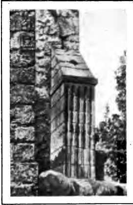
FIG. 107.—SAN MIGUEL DE LINO. ASTURIAN BUTTRESSES.
