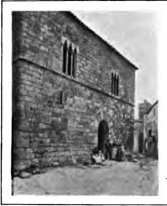
FIG. 273.—CASTELLON DE AMPURIAS. CATALAN HOUSE (14TH CENTURY). (Phot. of the Catalan Institute.)
