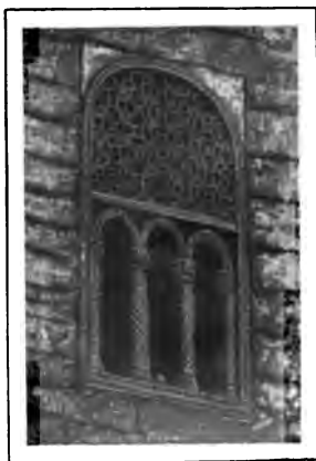
FIG. 116.—SAN MIGUEL DE LINO. AJIMEZ OF RIGHT TRANSEPT. (See Fig. 112.) (Author's Phot.)
