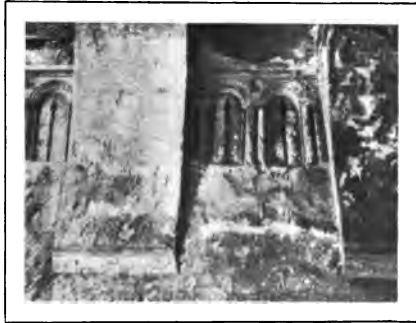
FIG. 54.—CASTLE OF EL OKHAIDHER. VAULT, INTERIOR ( comp. Figs. 25, 29).
