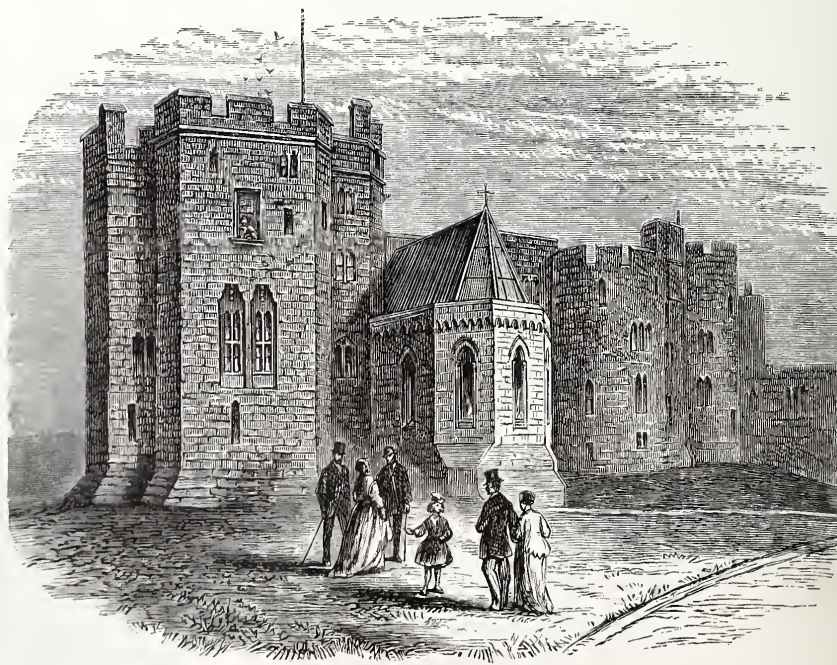
THE PRUDHOE TOWER AND CHAPEL.
