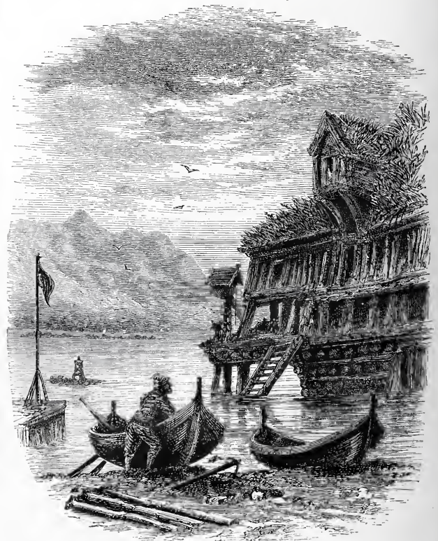
Sea Warehouse, Molde.
