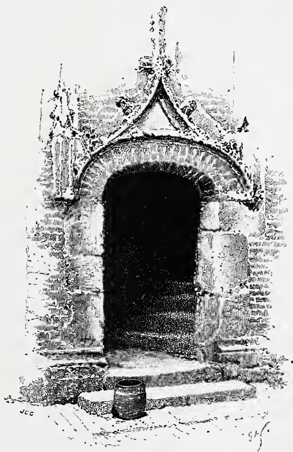
Courtyard Door, House of Tristan l'Hermite, Tours.
