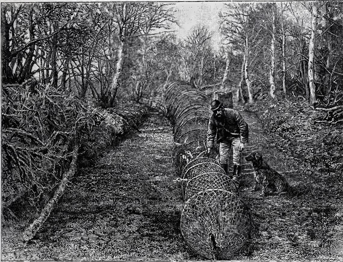
End of Pipe.
