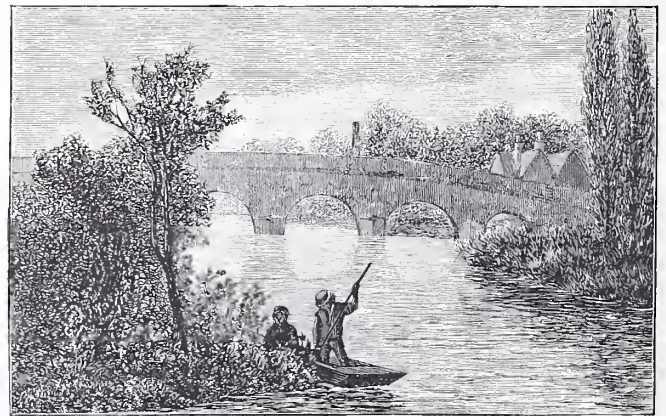
No. 28.—Chertsey Bridge.
