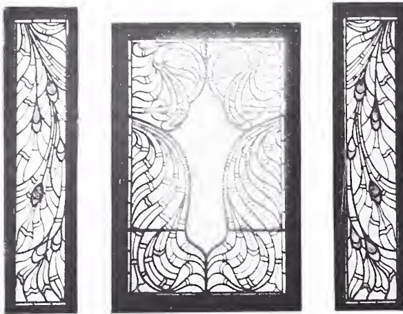
PANELS OF GLASS SHOWING THE EFFECT OBTAINED BY USE OF COLOURED GLASS AND LEADS ONLY. BY MESSRS. GUTHRIE, OF GLASGOW. (6.)
