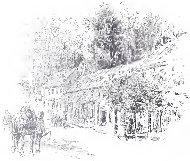
A bit of Bell Street, Reigate.
