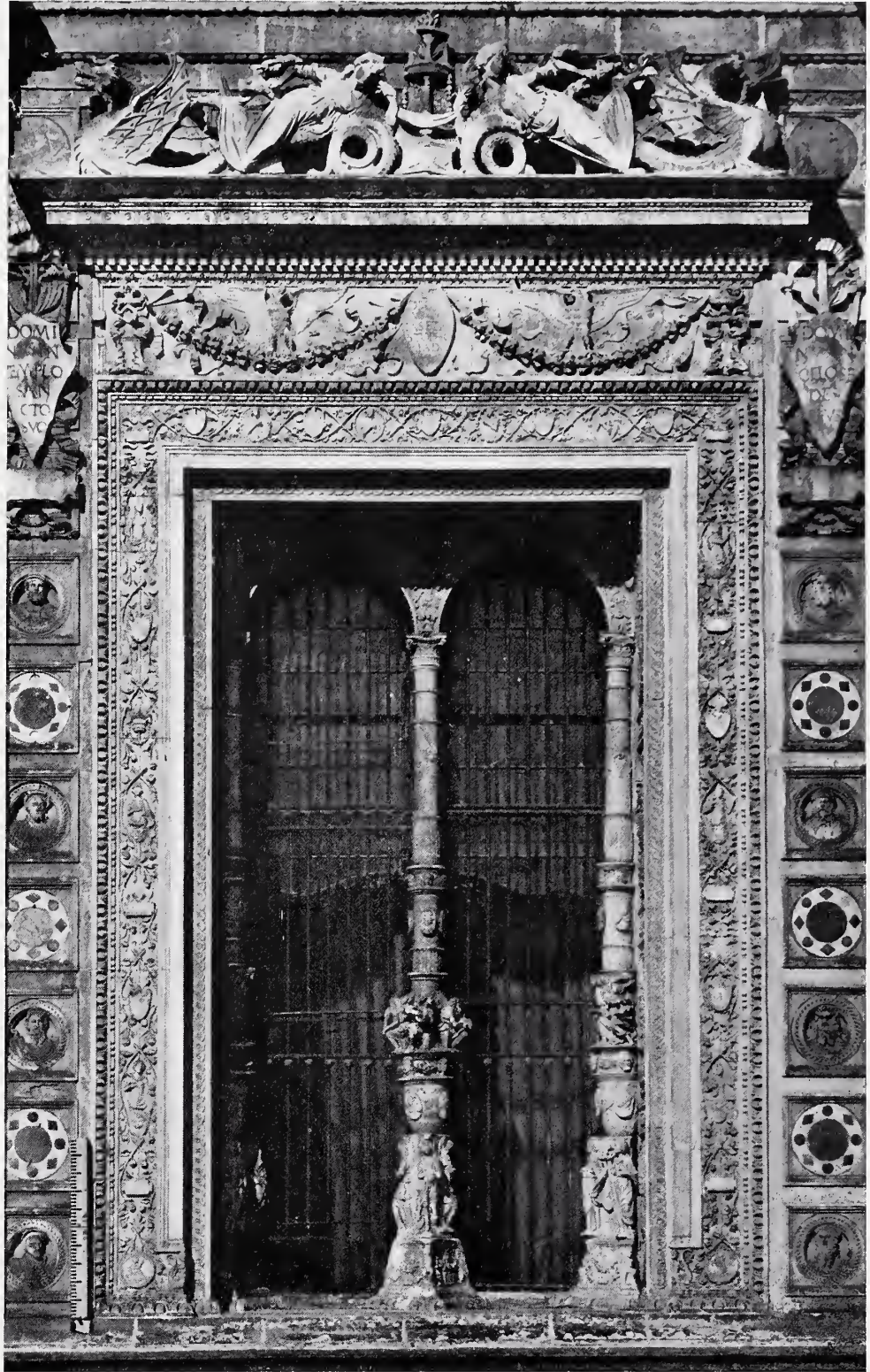
Window in the Façade.
