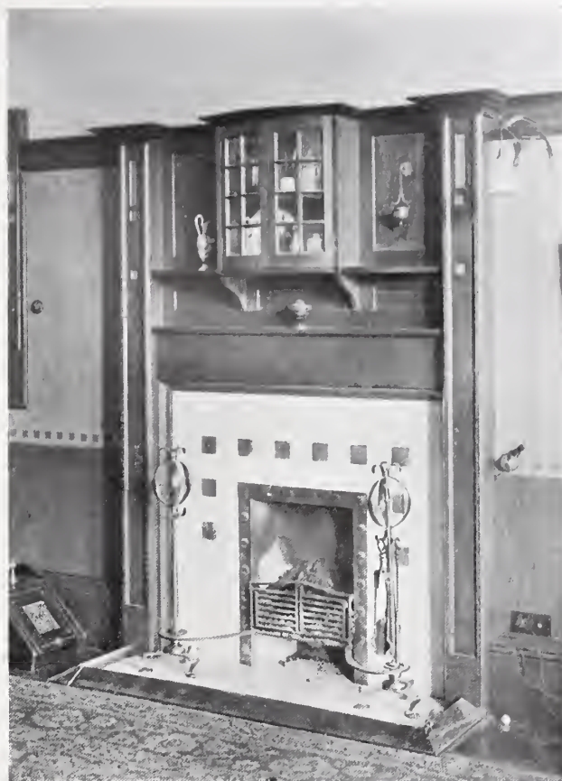
Dining-Room Chimneypiece in yellow pine, stained and varnished. Inlay on pillars of opalescent green glass.
