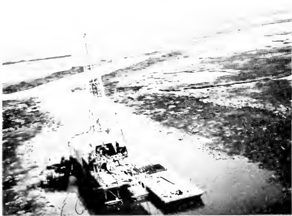
FIGURE 3.—An oil rig in the heart of the Louisiana marshlands. Eight-foot wide canals fanning out of main canals are dredged to accommodate barges ferrying-in oil rig equipment and support platforms. Photograph courtesy of Prof. W. D. McCain, Jr. of Mississippi State University.
