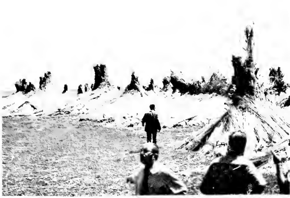
FIGURE 6. — Harvested stems of the common reed awaiting hauling by barges to the cellulose processing plant in Braila, Romania. Annually, approximately 120,000 tons of dry reed is harvested and processed yielding 60% dry pulp.
