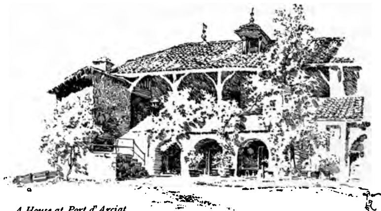
A House at Port d' Arciat.
