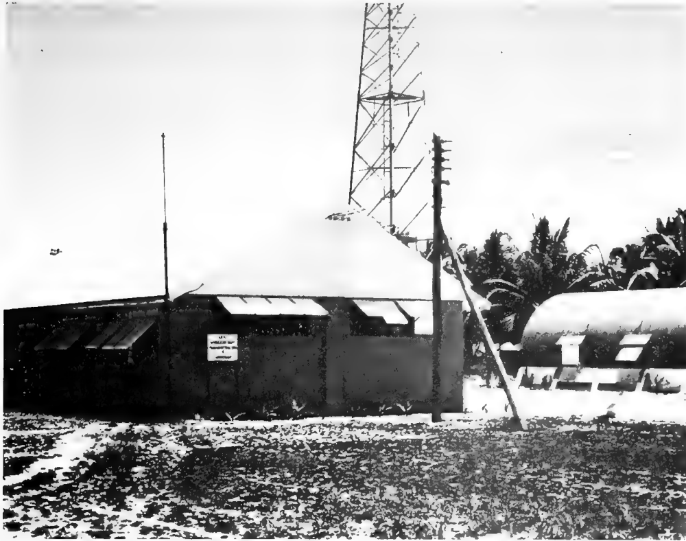
Figure 31. Transmitter Building at Betio.
