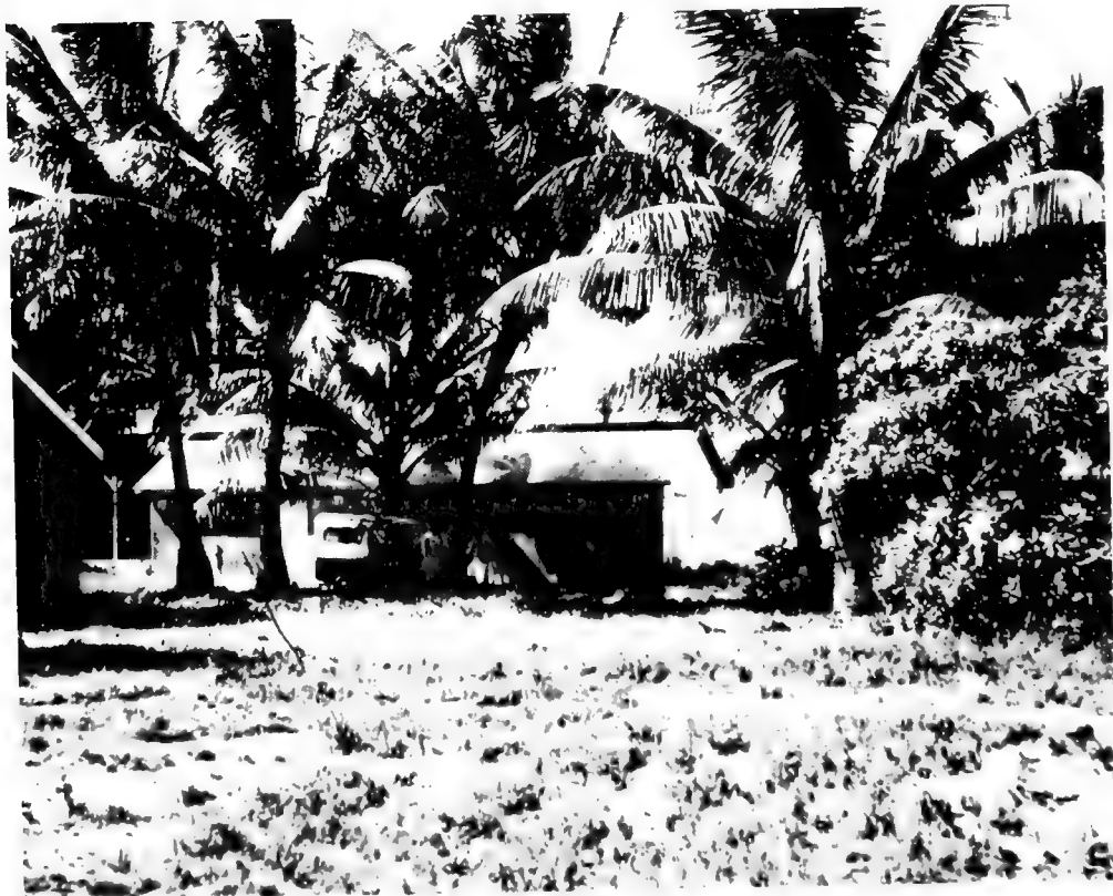
Figure 30. Buildings in Meteorological Station at Betio.
