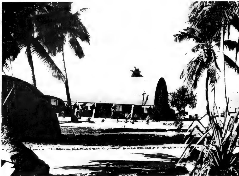
Figure 32. Nissen Building Used as Warehouse Near Dock at Bairiki.
