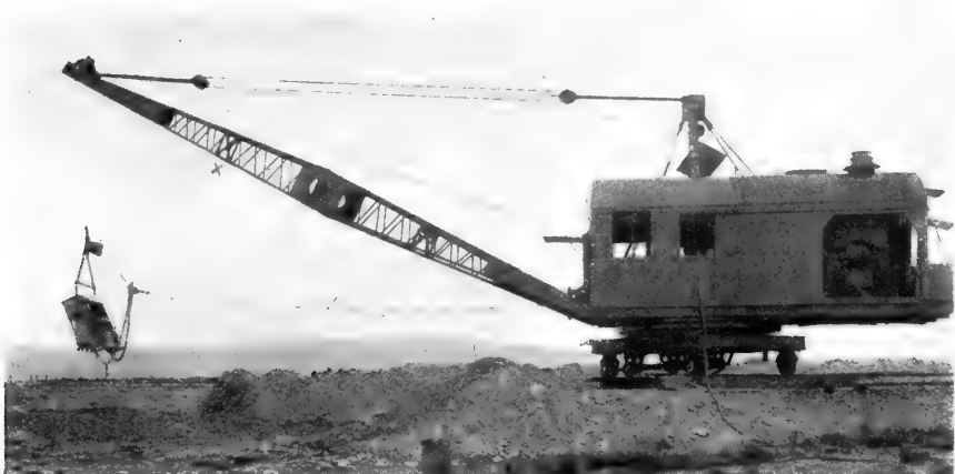
A PAIR OF FLYCATCHERS BUILT THEIR NEST AND REARED THEIR YOUNG AT THE PLACE MARKED X IN THE ARM OF THIS DREDGE WHILE IT WAS IN OPERATION
