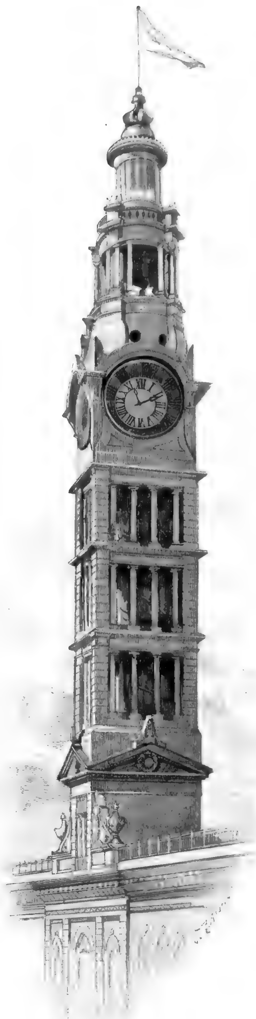
THE SYDNEY POST OFFICE TOWER.
