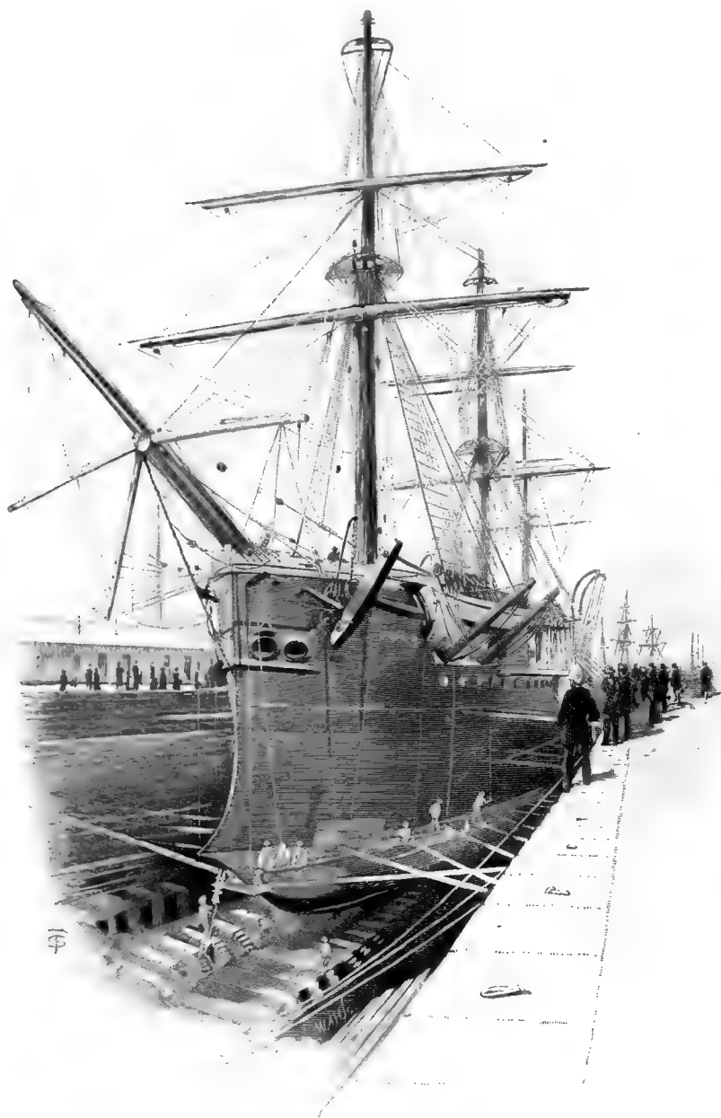
THE ALFRED GRAVING DOCK.
