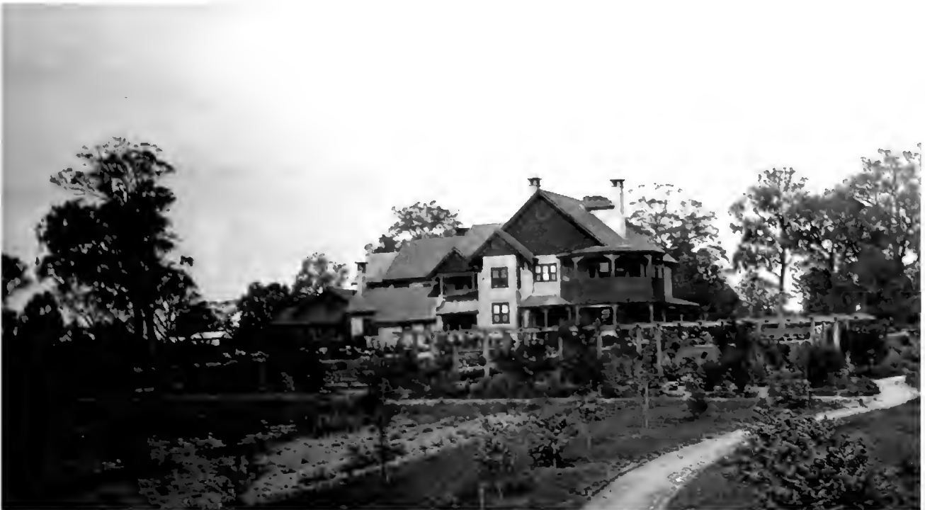
A broad view towards the house and garden from the north west (pre-1920). The wooden pergola is on the site of Joan Law-Smith's crab apple walk. Immediately in front of this are the lime trees ( Tilia sp.) which today form the boundary between the garden and the park. A serpentine path winds past the orchard to intersect with the poplar walk (see pages 6–7). Remnant trees from the Syme's orchard remain and recently new trees have been added, propagated from budwood taken from the survivors.
