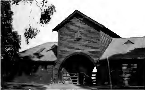
In his diary for May 1913, Syme noted the commencement of the erection of the 'Draught Stable'. Complete with stone floors the horses were housed on one side of the arch with the sulky stored on the other.
