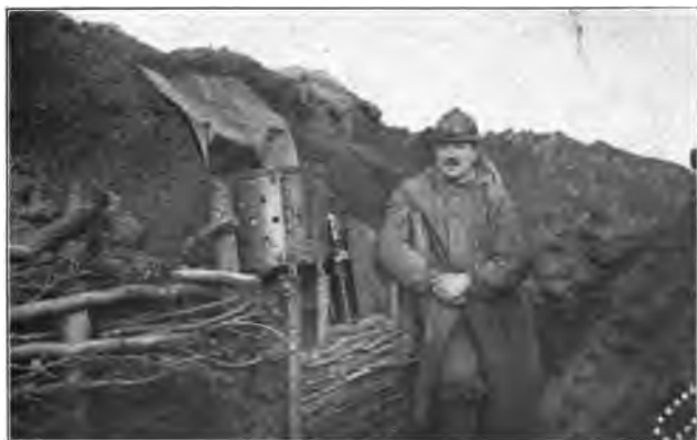
READY FOR GAS—A BRAZIER AND A BOTTLE OF GASOLÈNE. Hot air causes the gas to ascend
