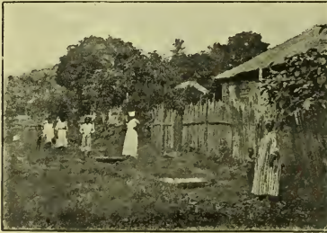
2. Street in Freetown, showing ditch at the side.
