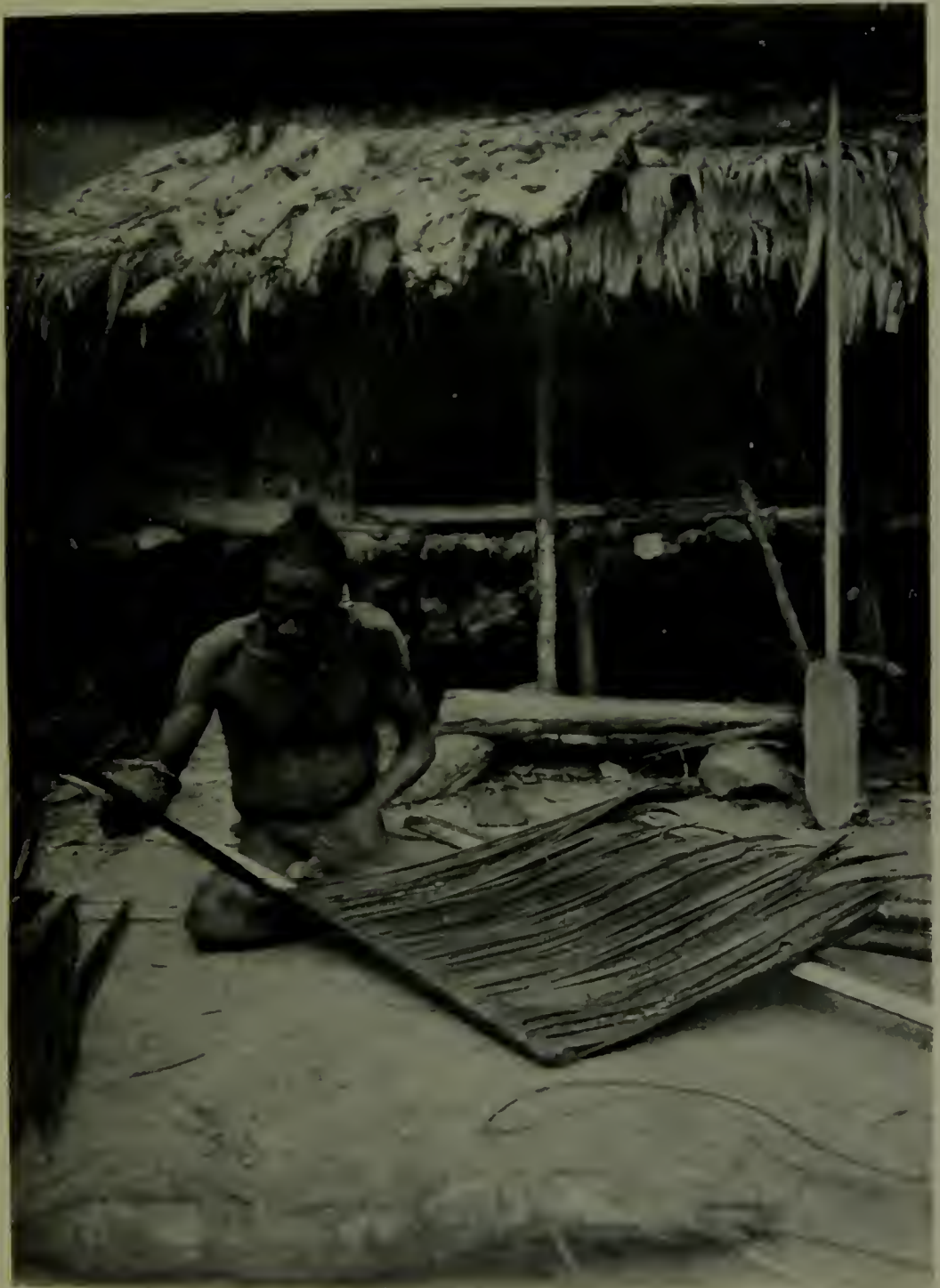
MAKING " ATAP " FOR ROOFING.
