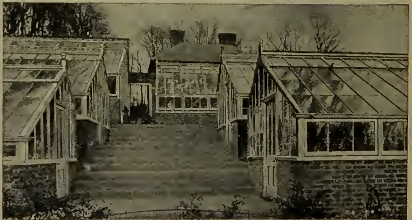
ERECTED AT OXTED, SURREY.
