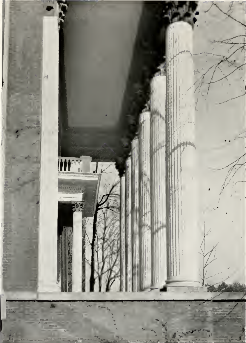
SIDE VIEW OF ADMINISTRATION BUILDING
