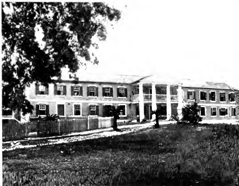
FIG. 2.—VIEW OF HOSPITAL, NASSAU
