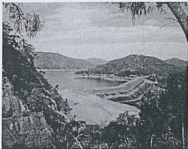
Lake Eildon wall being raised
