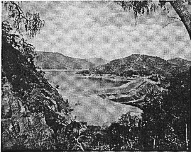
Lake Eildon wall being raised
