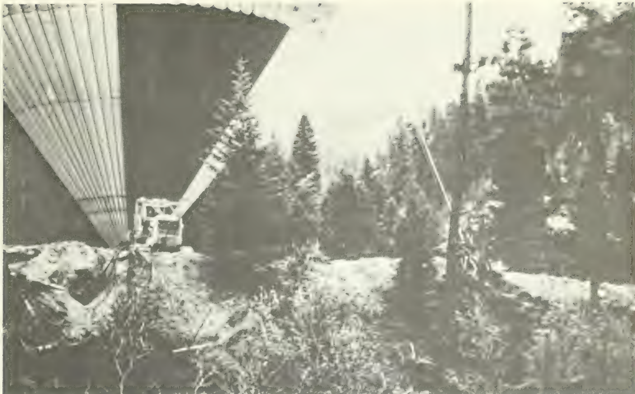
Figure 6.--Balloon bedding area in the Cow Creek subdrainage as it appeared shortly after construction.
