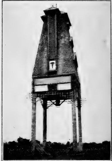
FIG. 4.—Bat roost near Military Academy, San Antonio, Tex., built by popular subscription in 1920 at a cost of $2,000, for mosquito control, but never occupied. In only one of eight such structures, from Florida to Texas, have bats taken up their abode
