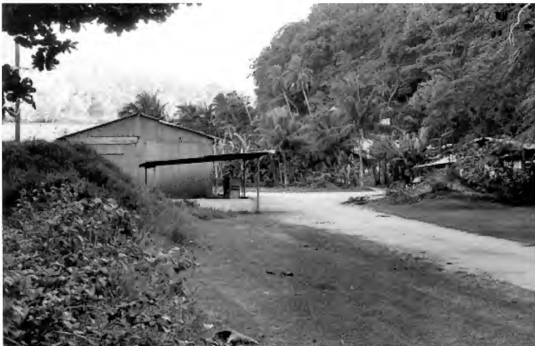
Figure 80. Photograph of some of the buildings in Duanvale, Trelawny Parish, Jamaica, from which Molossus molossus were observed exiting.
