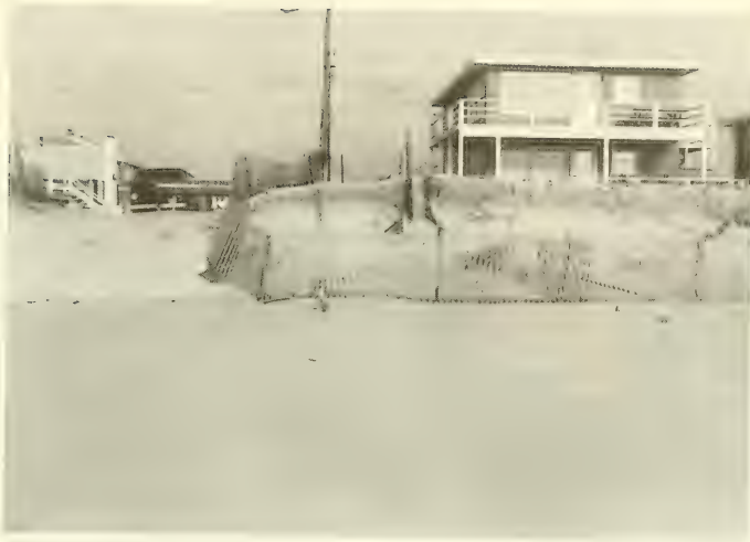
c. Typical beach access through dunes at profile line 15. Such locations were washover sites during the March 1962 storm.
