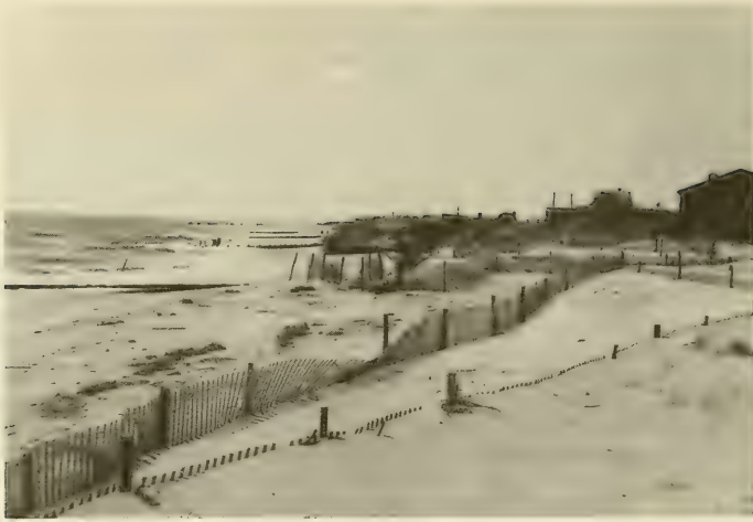
a. View looking south from profile line 1, showing extensive sand fencing, groins, and development.
