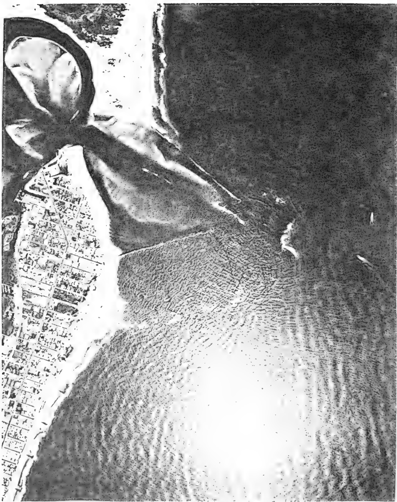
Figure 3. Air photo of Barnegat Inlet and converging jetties. Note the confused wave refraction over the shoal south of the south jetty.
