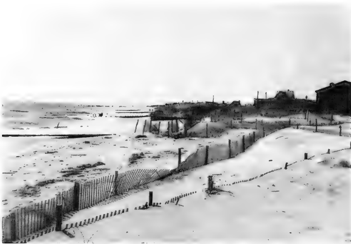
a. View looking south from profile line 1, showing extensive sand fencing, groins, and development.
