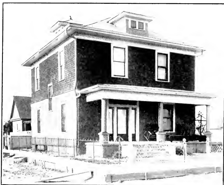
RESIDENCE OF WILLIAM BURROWS. Contractor and Builder
