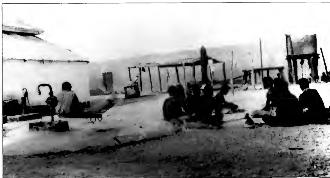
Fig. 3. Photograph of subterranean tank in Area A, looking toward eastern perimeter fence. Note concrete lid, pumps, drainage channel and washstand and tub (in background). Photograph of unknown date but almost certainly within the period 1910-1930s. (Photo: Museum and Art Gallery of the Northern Territory).
