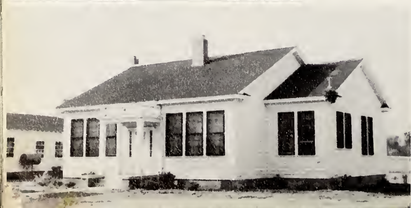
Landscaping project begun
