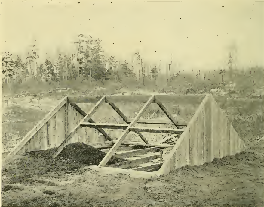
Covering the Floor with Sawdust Before Putting on the Roof.
