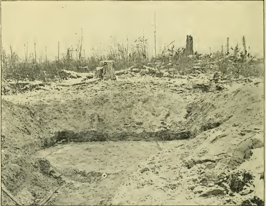
One Day's Work, Plowing, Scraping and Digging.
