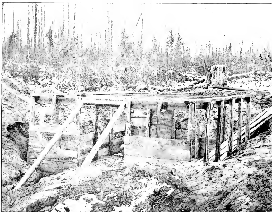
Putting up the Frame and Boarding up the Sides.
