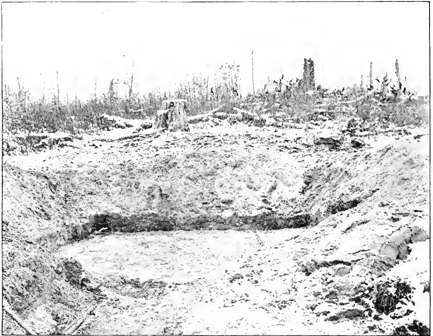
One Day's Work, Plowing, Scraping and Digging.
