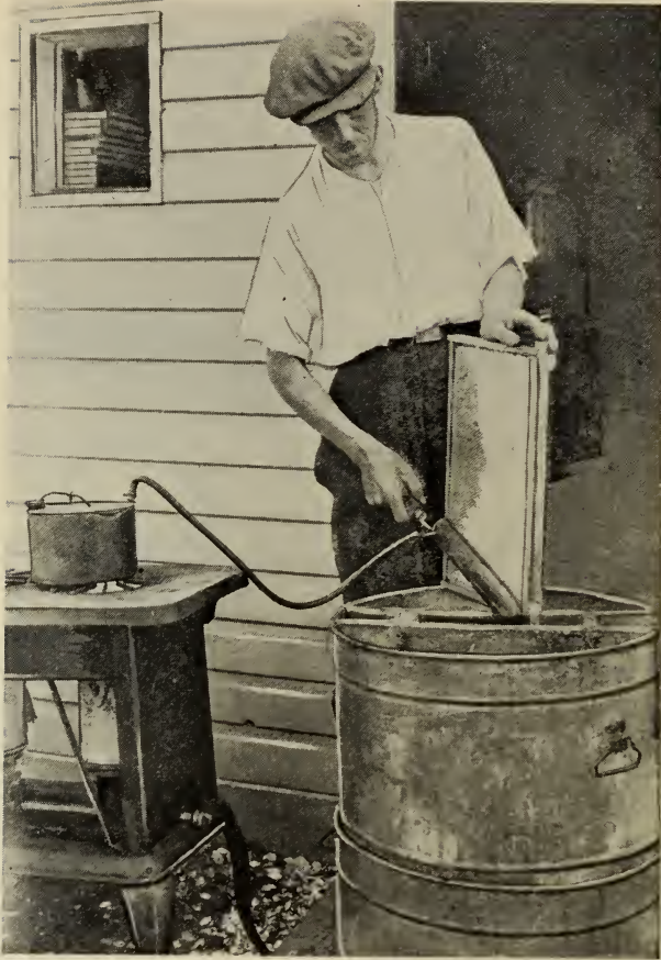
FIG. 23.—Uncapping comb of honey with steam-heated knife.
