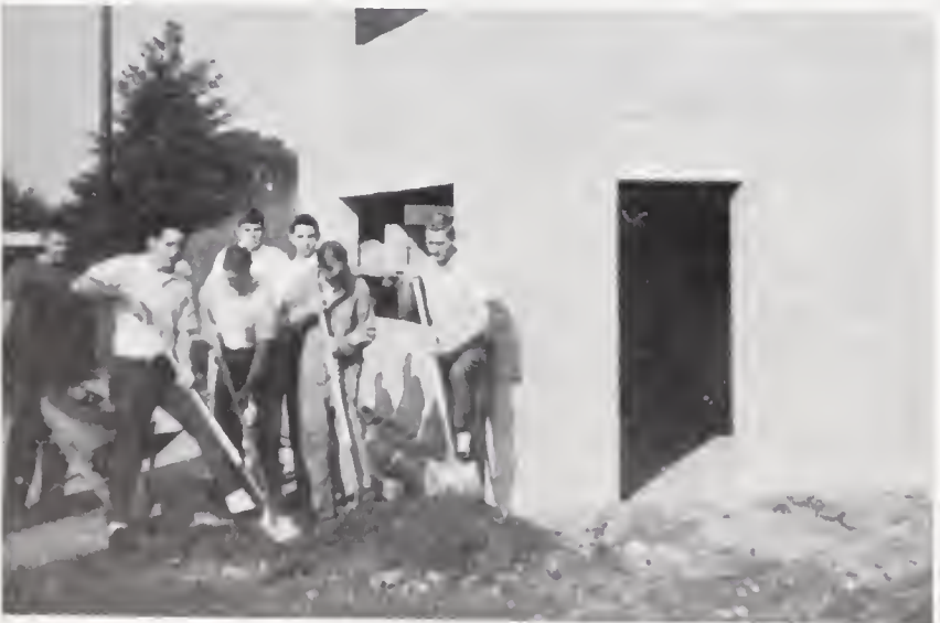
Building a new concession stand
