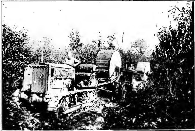
Fig. 12—Tractors Placing Cable Reels in Rough Country
