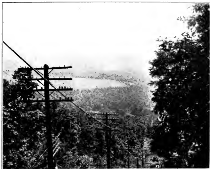
Fig. 8—Cable Line Across Valley at Grand View
