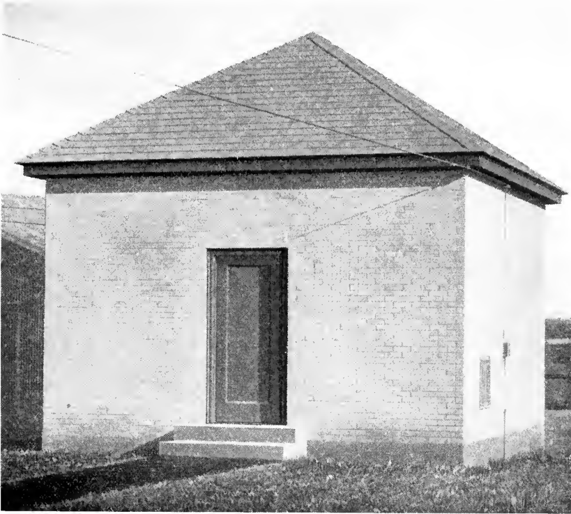
Fig. 12—Unattended repeater station.
