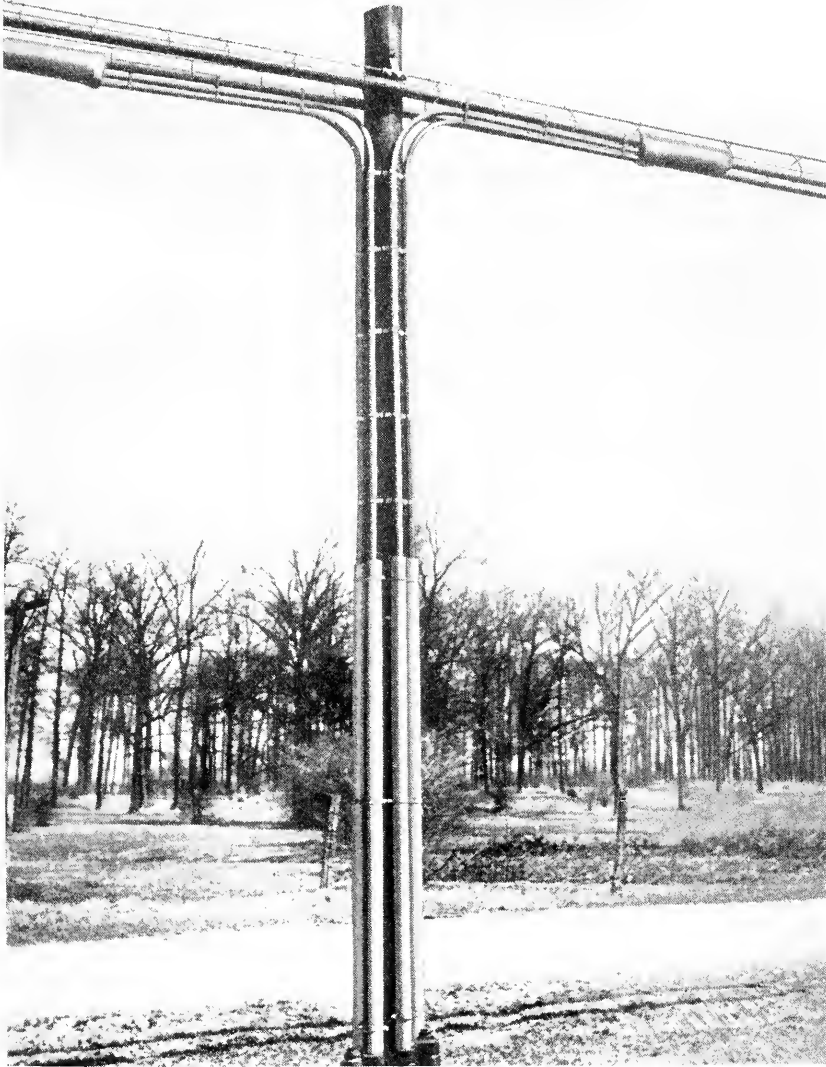
Fig. 4—The four lateral cables containing carrier pairs shown as installed at an auxiliary repeater point on aerial cables.
