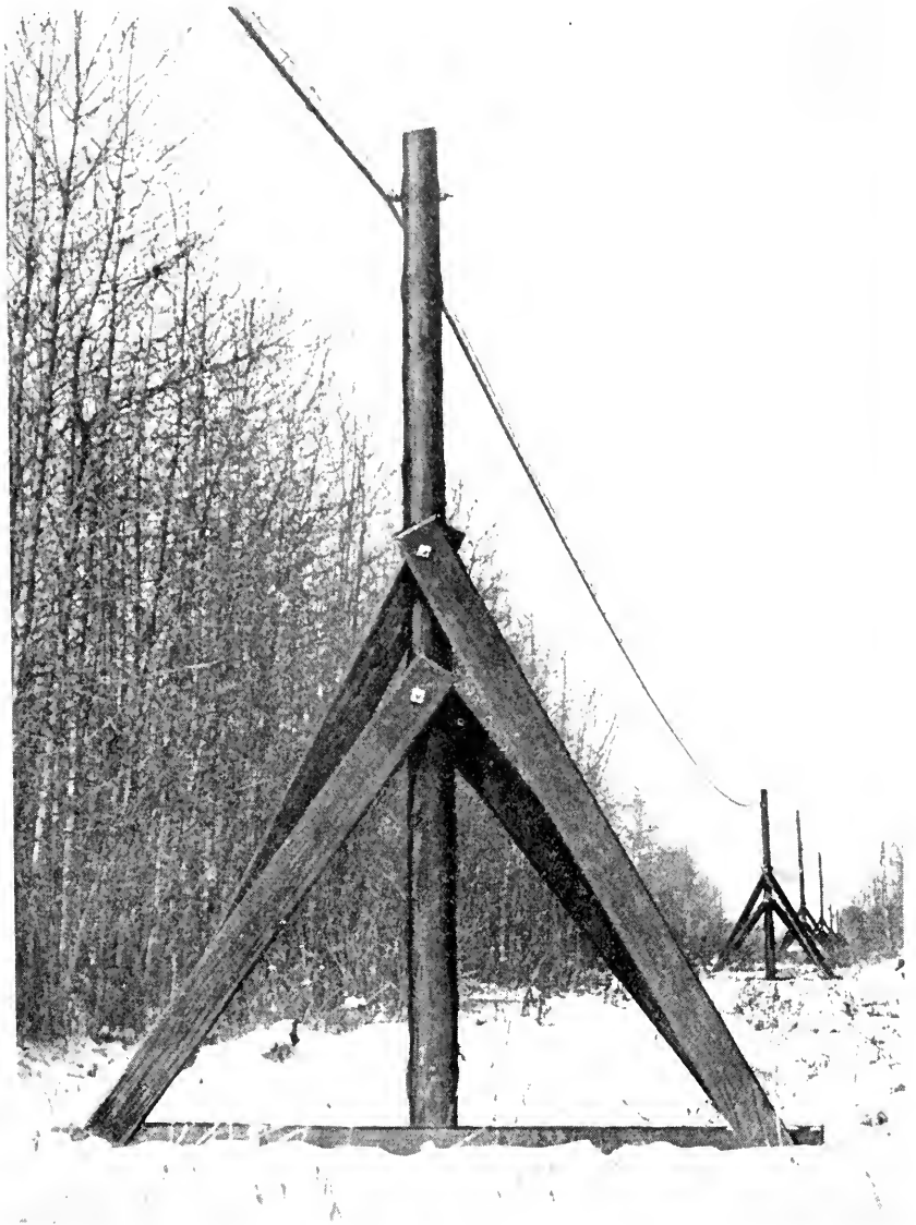
Fig. 3—Swamp construction.
