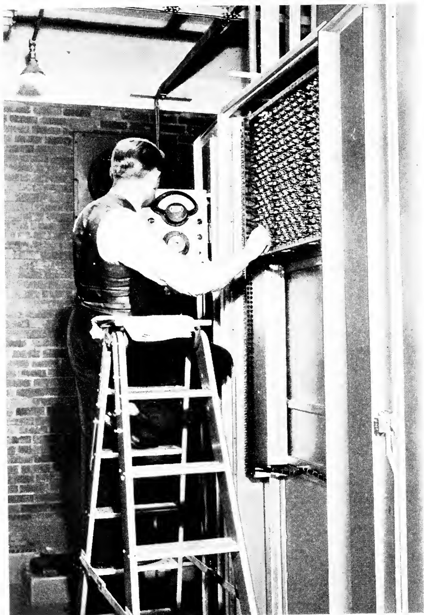
Fig. 3—Adjustment of coils in crosstalk balancing panel.
