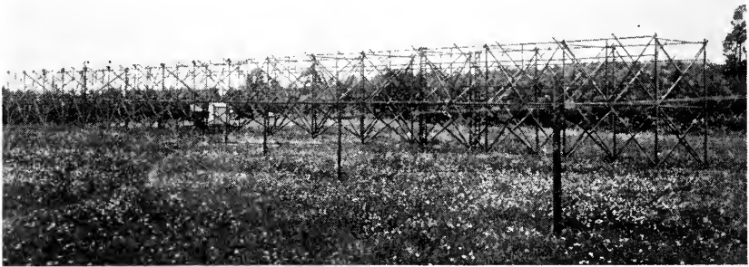
Fig. 18—Bruce receiving antenna at Netcong, New Jersey, used for transoceanic communication. This type of antenna has been superseded by the rhombic type at Netcong.
