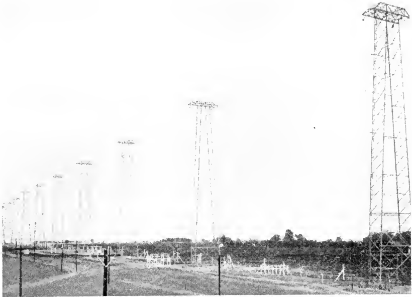
Fig. 16—Towers at Lawrenceville, New Jersey, used to support a number of Sterba antennas for transoceanic communication. These antennas have since been superseded by rhombic antennas.
