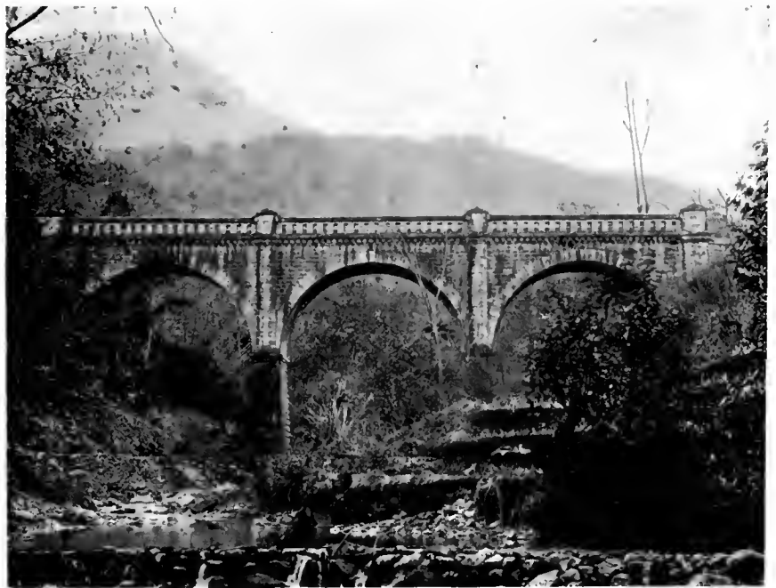
A FINE STONE THREE-ARCH BRIDGE
