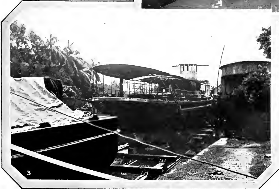
2. TWIN-SCREW STEAMER, 110 FT. X 17 FT., AND CARGO-FLAT, 150 FT. X 26 FT., UNDER CONSTRUCTION ON SLIPWAY.
