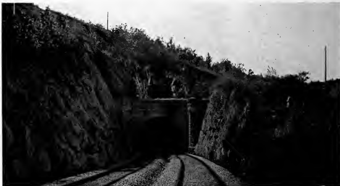
A TUNNEL ON THE GRAND CHORD, EAST INDIAN RAILWAY.
