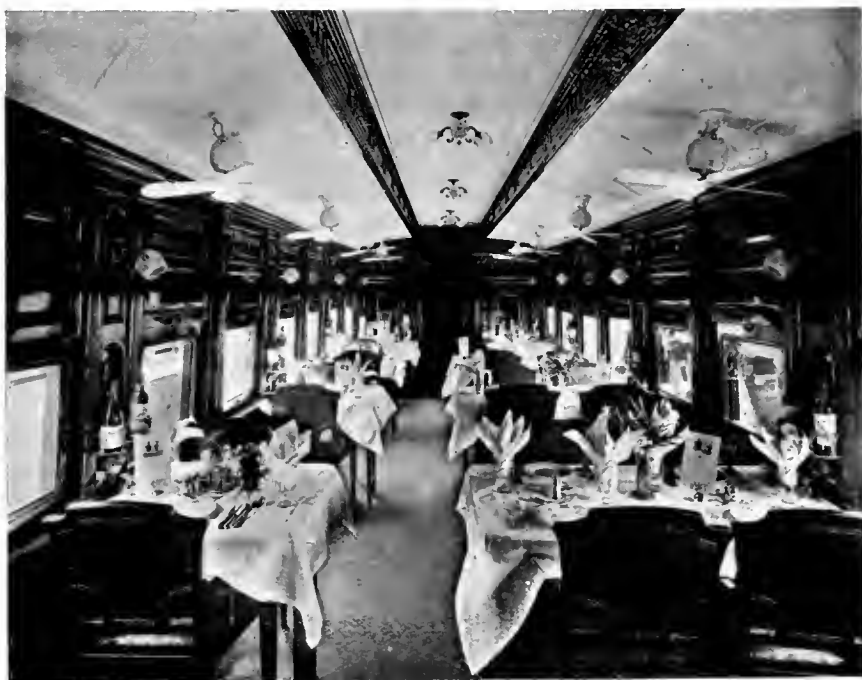
INTERIOR OF A BENGAL-NAGPUR RAILWAY REFRESHMENT CAR.
