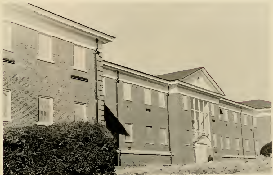
The New Science Building
