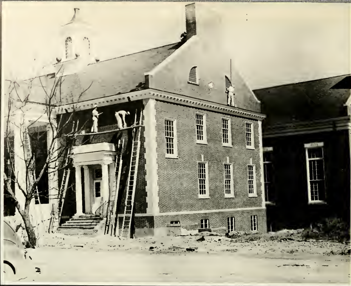
Construction of the David D. Jones Student Union
