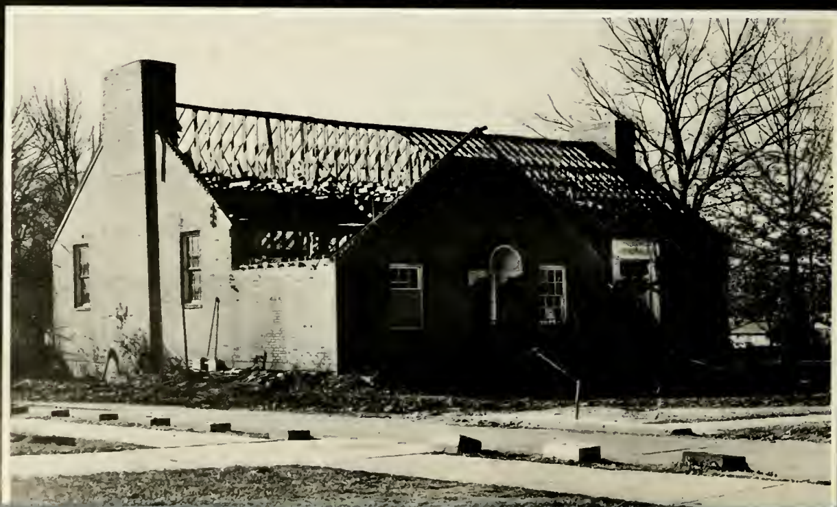
Demolishing the Thurkfield Gym — 1913
