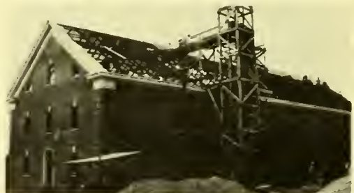
Pfeiffer Hall under construction.
