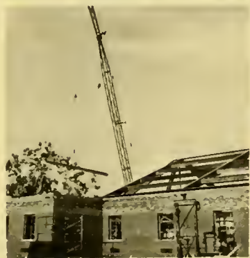
Construction of Pfeiffer Science Hall (1967)
