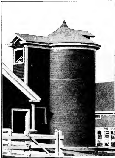
THE WOOD WRAPPED SILO A good type of modern silo.
