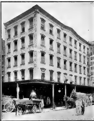
Five Stories and Cellar Corner Harrison and Washington Streets.
