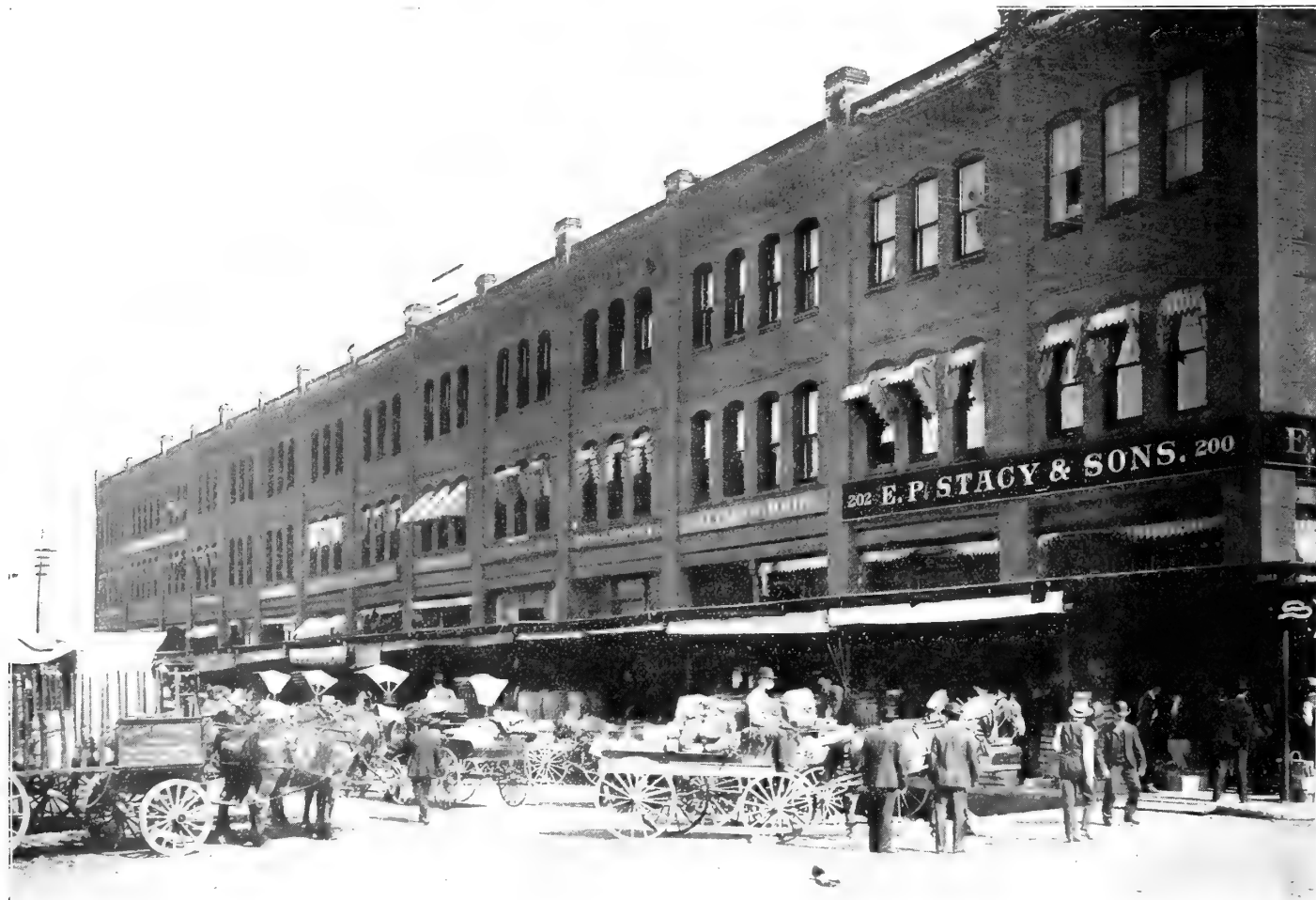
COMMISSION DISTRICT, MINNEAPOLIS, MINNESOTA, SHOWING E. P. STACY & SONS AT CORNER. List of their branch houses is given in their advertisement in this edition
