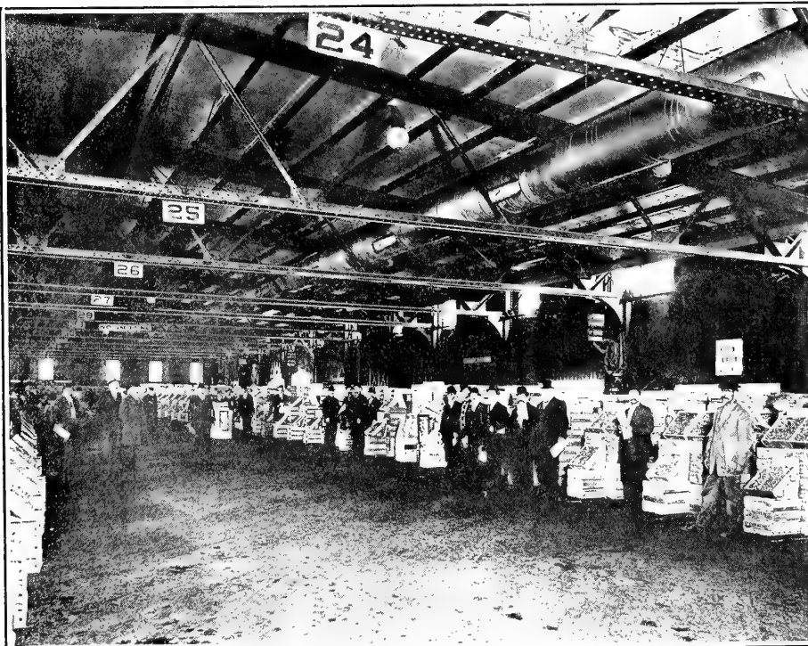
VIEW OF THE ERIE DOCK, NEW YORK CITY
