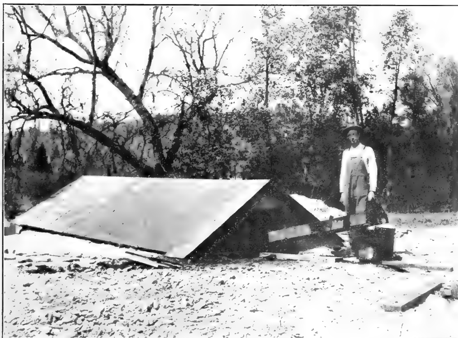
Figure 9—Pritchard Orchard, Grants Pass, Oregon. Crude Oil Storage Tank
