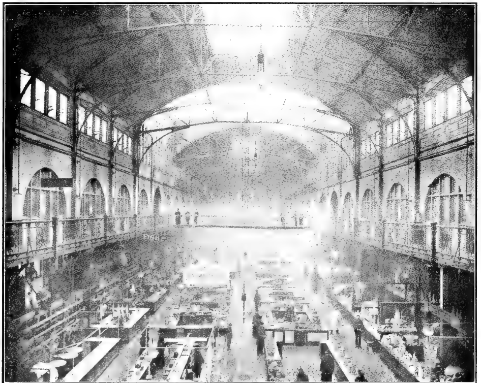
INTERIOR VIEW OF MARKET HOUSE—SHERIFF STREET MARKET AND STORAGE COMPANY, CLEVELAND, OHIO
